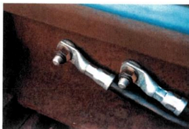
AR60D rail web connections - rail side
