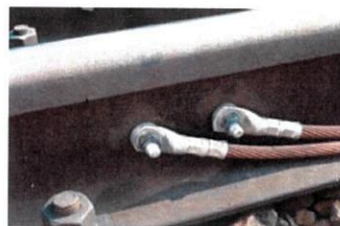
Example of connections using a low stranded conductor to provide electrical continuity on cast manganese steel crossovers
