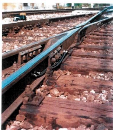
Example of connections using a flexible cable to provide electrical continuity on cast manganese steel crossovers
